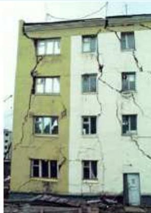
A railroad in Alaska (left) and building (right), both buckled due to thawing permafrost.
